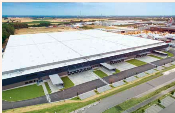
INTERPARK – EINSTEINSTRASSE Completed in 2015, Rental area 55,000 sqm
