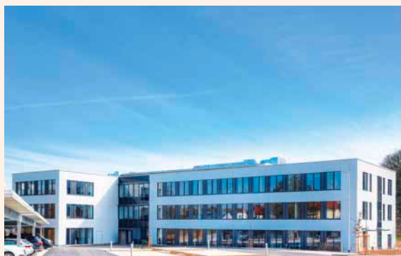
VIB HEAD OFFICE IN NEUBURG/DANUBE, Completed in 2017, Rental area 2,700 sqm
