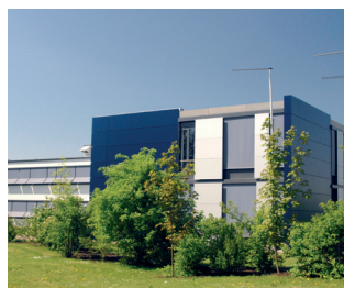
Production and office building, Neuburg/Donau
