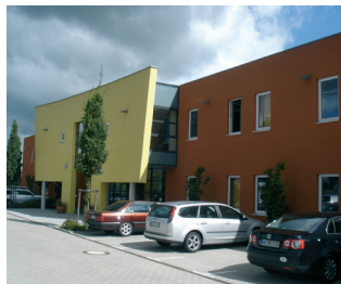
Production and storage building, Heroldsberg
