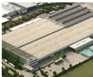
Production and logistics hall, Neufahrn
